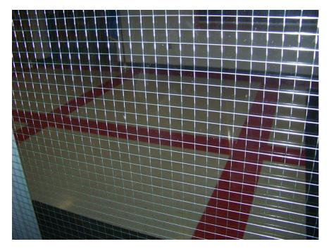
This type of glass is the best type to use because the only way through it is with an ax. The fire departments don't usually like this glass but it holds up great to most bullets.
