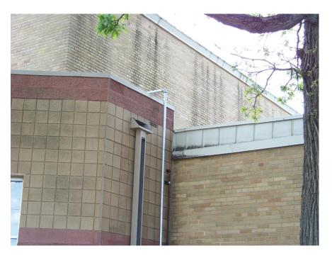
Install some type of cone safety device on the gas line for the pool so that it will limit someone to use the gas line as a way onto the entire building roof.
