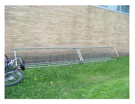
Install a concrete pad to anchor the bike rack securely to the ground. We don't want anyone propping the bike rack up on the side of the building and using it as a ladder.
